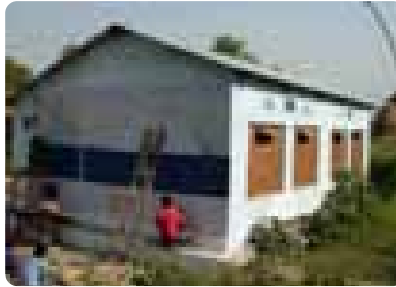
▼ An emergency shelter at Prasauni, Chitwan.
