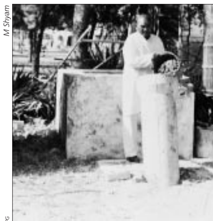
Figure 5: Pouring fresh cattle dung straight into the feed pipe of the plant
