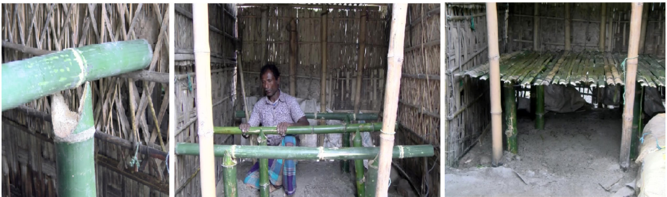
Photo 3 Construction of bamboo raised platform
