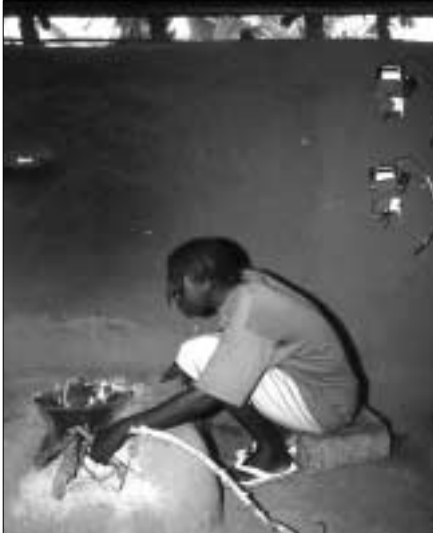
Figure 3 Eaves spaces and Upesi stove installed in West Kenya (photo: Nigel Bruce)
