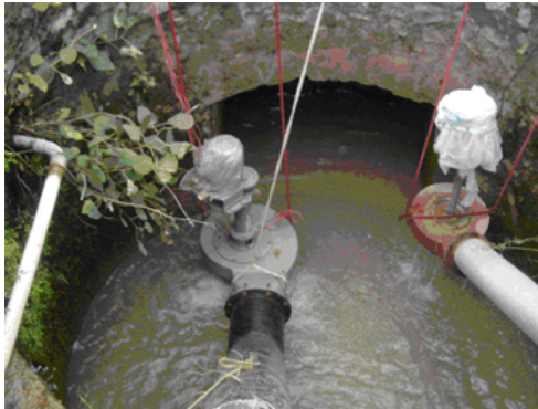
1 & 2 kW Pico Type Kaplan Turbines working on 1.5 m head & Discharge 10 Cusecs
