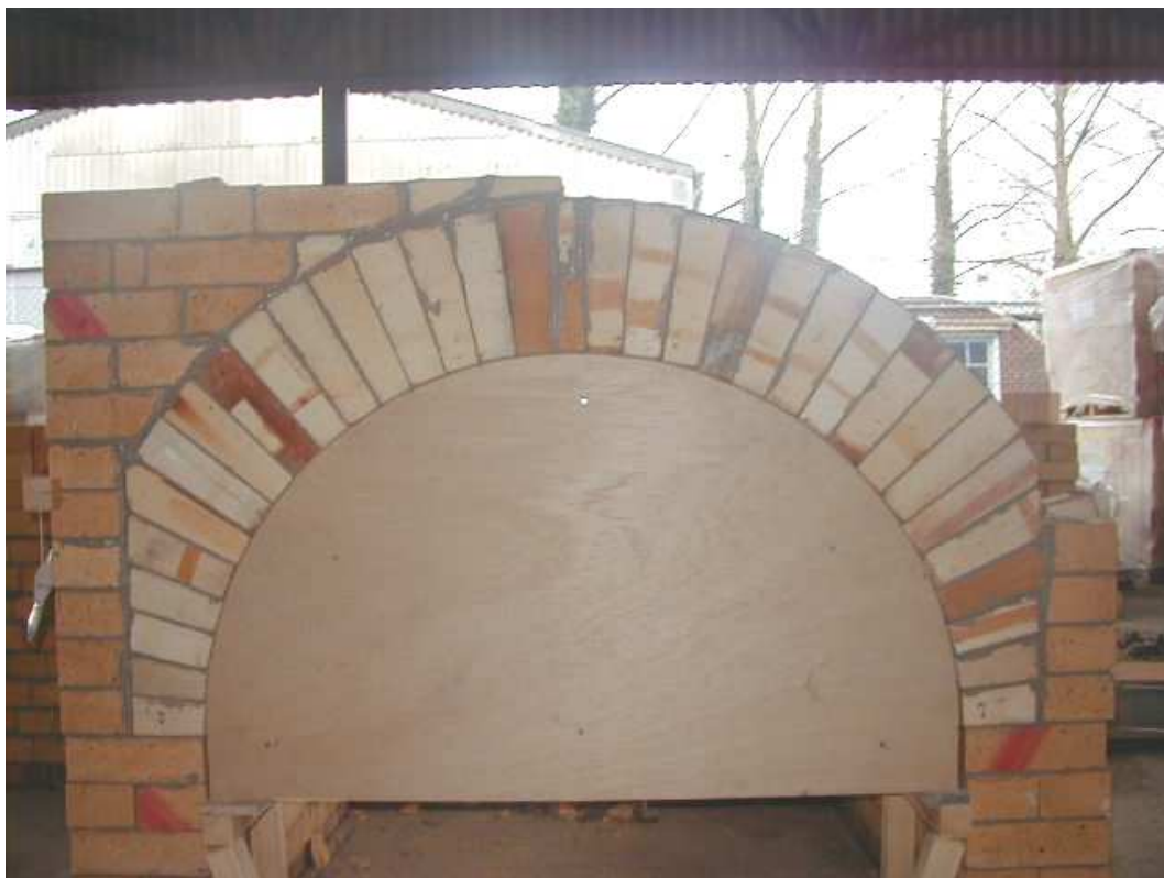
Figure 3.6: Primary chamber access arch construction (with former in place) from the Ash End
