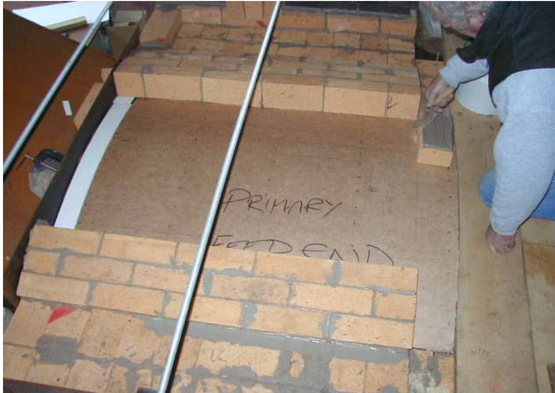
Figure 3.12: Primary chamber arch under construction.
