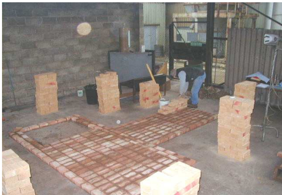
Figure 3.3: Laying refractory bricks (from stack end)
