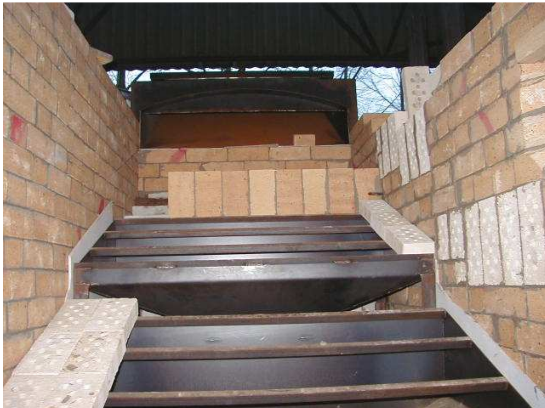
Figure 3.5: Perforated refractory bricks being laid on plenum/grates
