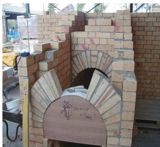
b: Access arch
