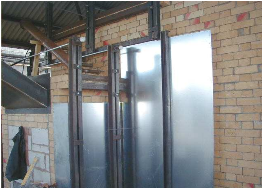
Figure 3.17: Sheet steel retaining wall under construction
