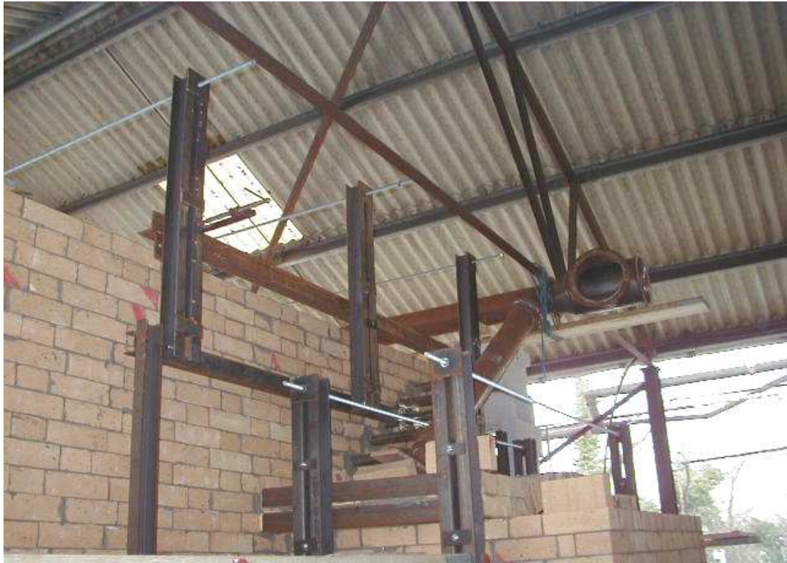
Figure 3.15: Secondary chamber buckstay frame and backstays in position
