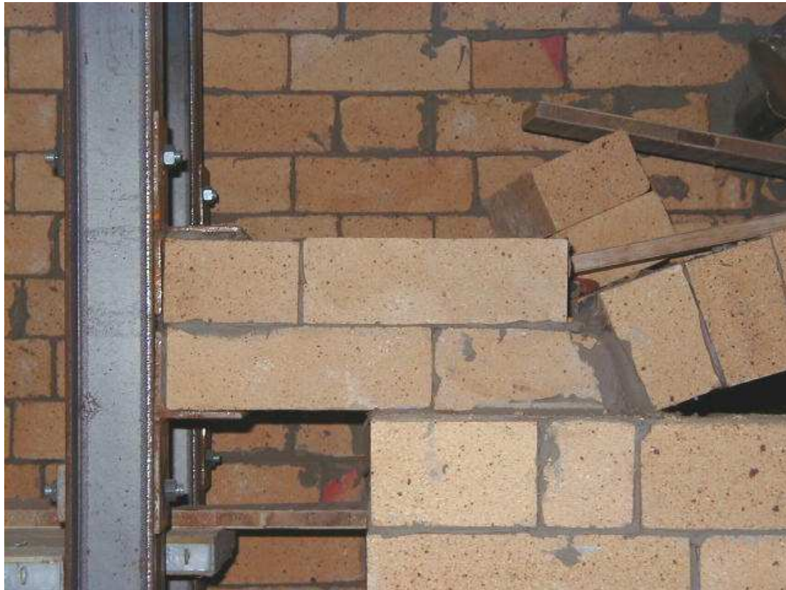
Figure 3.10: Skew-brick and skew-brick rails in position.
