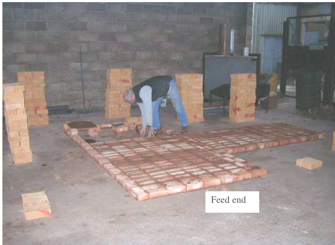
Figure 3.2: Laying LCI floor
