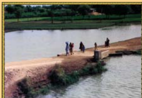
Culvert providing protection from floods and mobility to villagers during the monsoons
