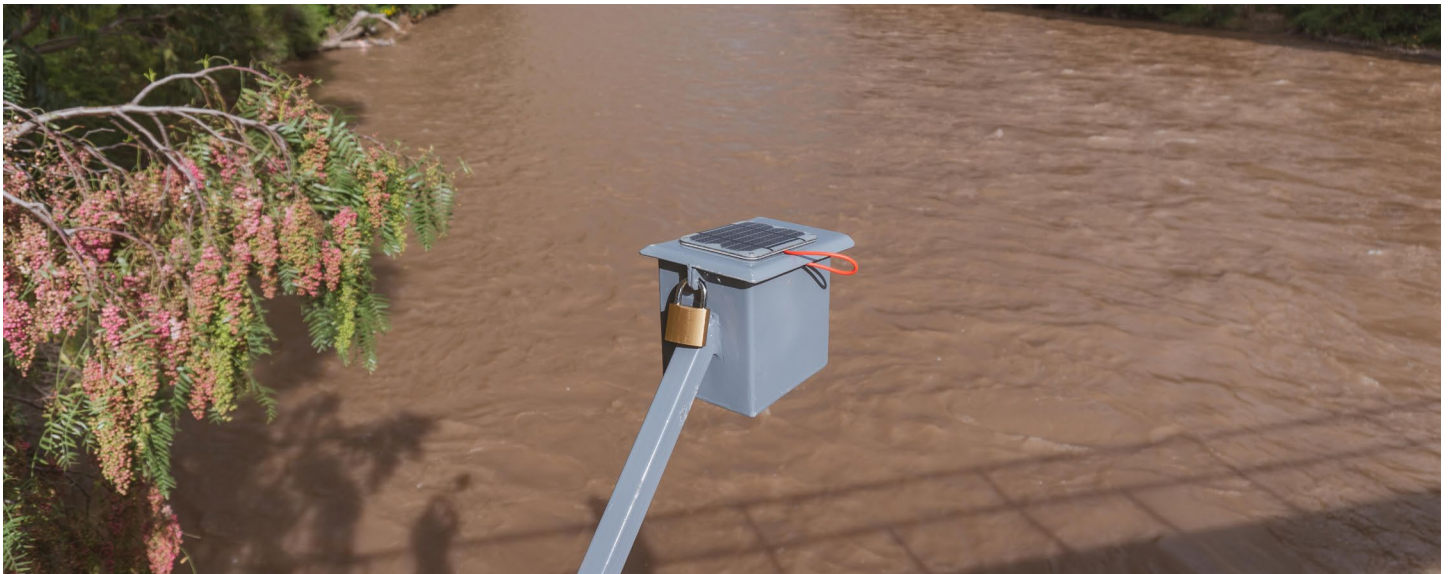
Hydrological monitoring station using lidar technology with metallic protection cover in the Vilcanota basin, Cusco, Peru, 2022. Giorgio Madueño (Practical Action)
