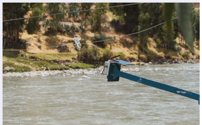
Hydrological monitoring station with lidar technology in the Vilcanota watershed with support structure, Cusco, Peru, 2022. Giorgio Madueño (Practical Action)
