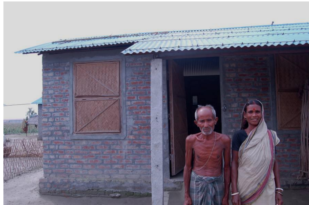
Figure 7: Husband and wife standing in front of their new house. Photo: Practical Action Bangladesh.
