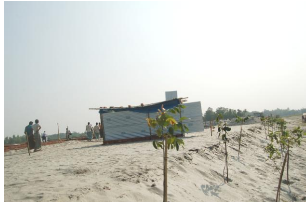
Figure 9: The newly finished earth raising is planted with young trees to stabilise the sandy soil. Photo: Practical Action Bangladesh.
