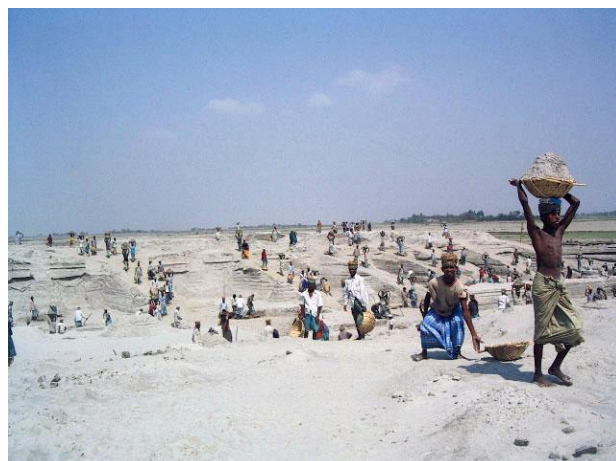
Figure 8: The whole community work together to make a large raised platform for the cluster village. Photo: Practical Action Bangladesh.
