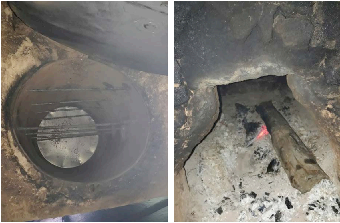
Figure 6.1 A close-up of the oven in Kigeme showing where bread is cooked (left) and the entrance to the firebox that fuel (firewood) is fed into (right)
