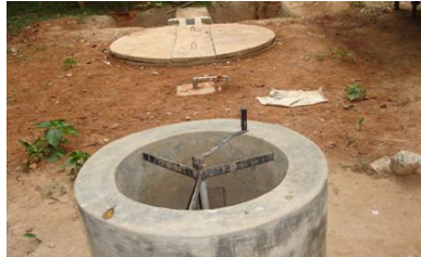
A Complete Plant (New)
