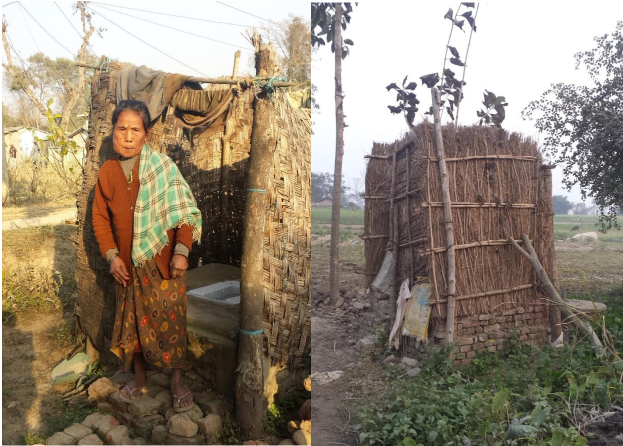
Photos: Simple technologies for superstructure to aid affordability
