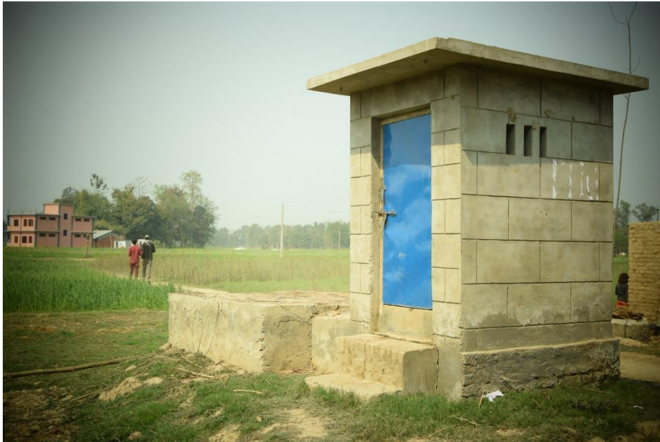
Photo: Raised, flood proof toilet.
