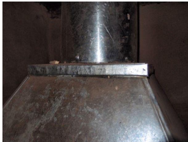
Figure 6: Detail of the metal fold at the hood intersection.
